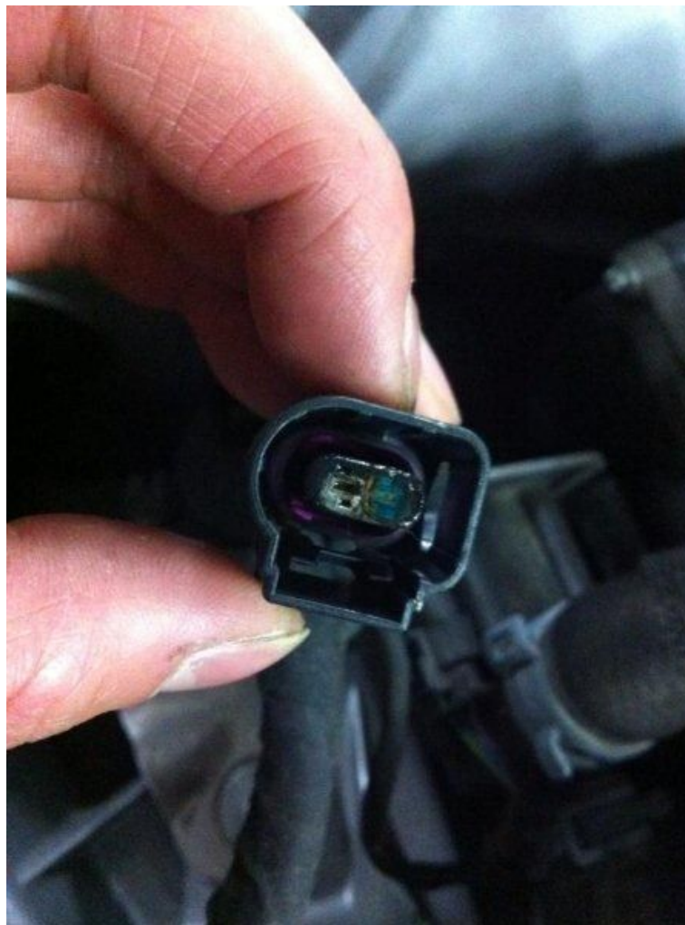
Figure 2. Corrosion formation on the connector pins.
