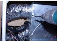
5. Remove the bottom and side screw from the furnace. Slide the furnace out of the cabinet.
