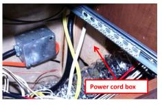
If there is a power cord box, no other action is required. If box is missing, proceed to Step 2.
