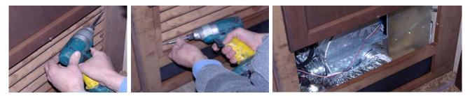
4. Loosen and remove the (4) heat hoses from the furnace.
