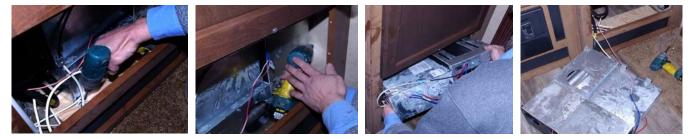
Insert the power cord box into the cabinet base. Using 1-1/2" screws, fasten the cleat on the top of the box to the bottom of the wardrobe shelf. Fasten the cleat on the bottom of the box to the rear wall. NOTE: recommend minimum of 4 screws per cleat.
