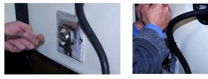
3. Remove the interior furnace grill by removing the screws on both sides of the grill. Set the screws and grill aside for re-use.
