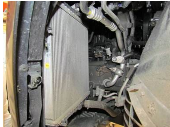
Figure 9. Charge air cooler exit air duct installed.
