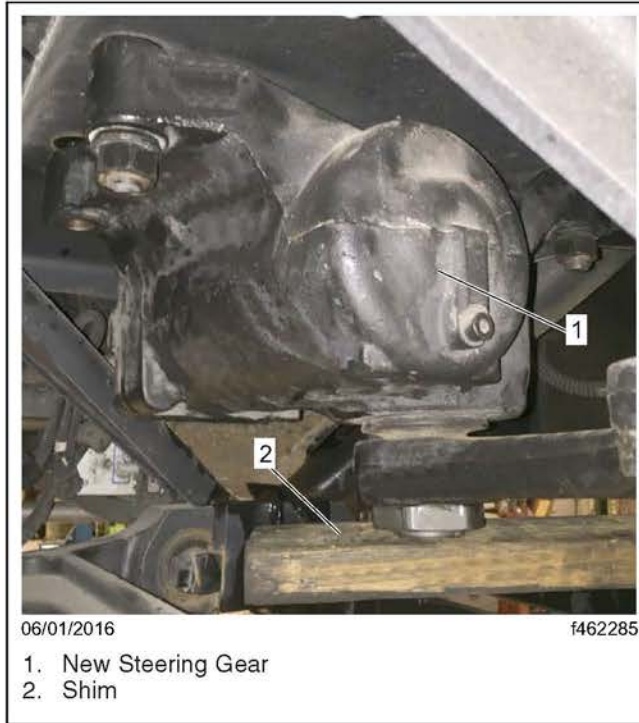
Fig. 14, New Steering Gear Installation
