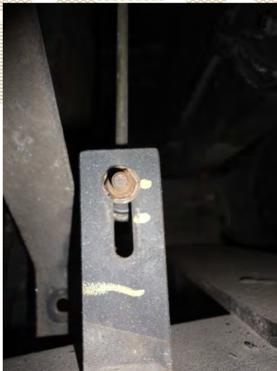
Figure 3 Marking Lower Link Bracket
