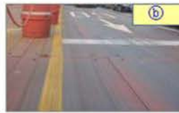
● Steel floor (subway construction site)
