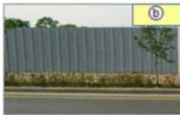
● Iron wall at the construction site
