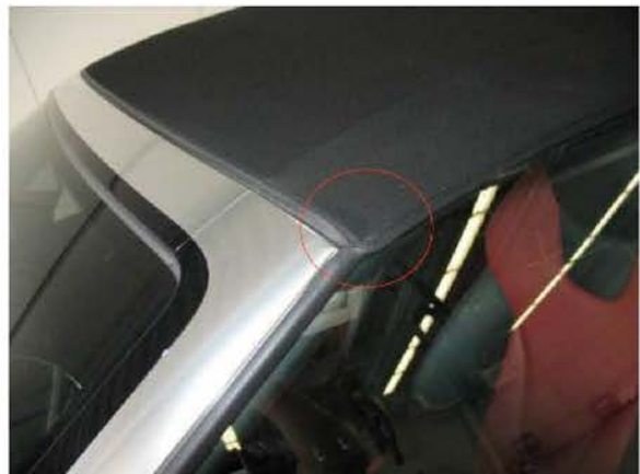
Figure 1. Location where a leak may occur.
